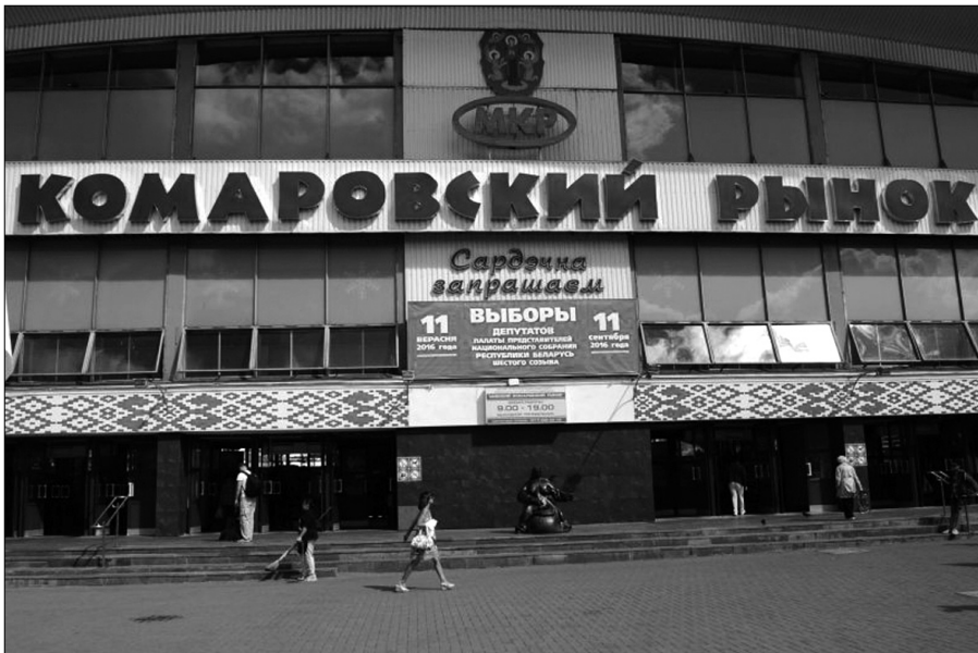
Information on the elections on the building of the Kamaroŭski market. Minsk, 25 August 2016
